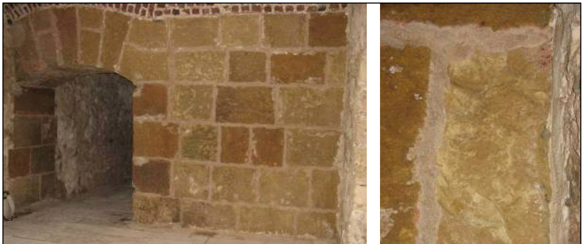
Figure 13 - foundation blocks made of (megascopically) yellowish to brownish sandy limestones.
